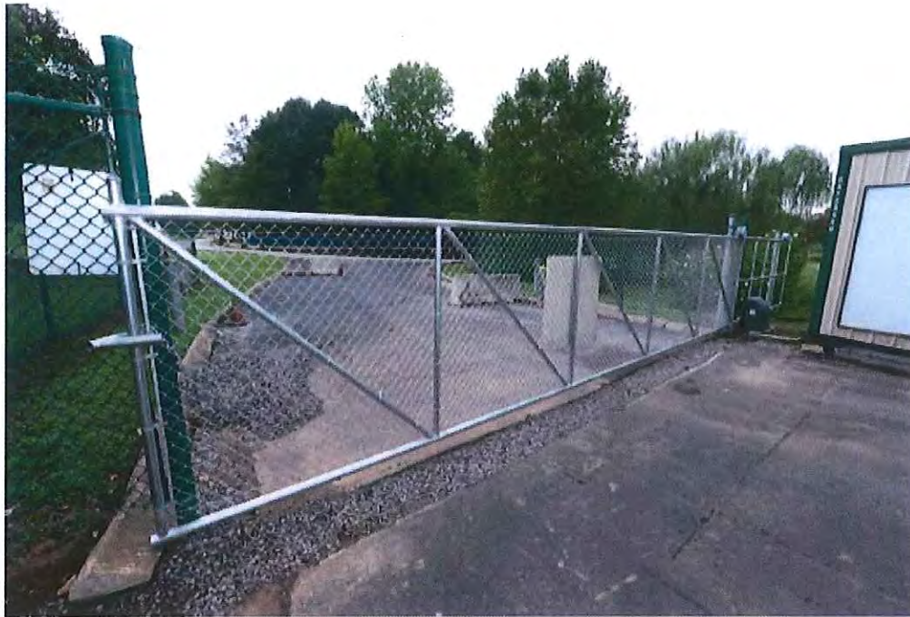
Photos taken by investigation team on August 19, 2015 showing repaired main gate and front entrance barriers at NOSC Chattanooga.
